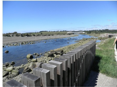
Water front walkway in New Plymouth New Zealand where sea washes over the natural timber, along with and continuous salt spray attacks the timber as shows signs of dry rot, splitting, and general corrosion to fittings.
