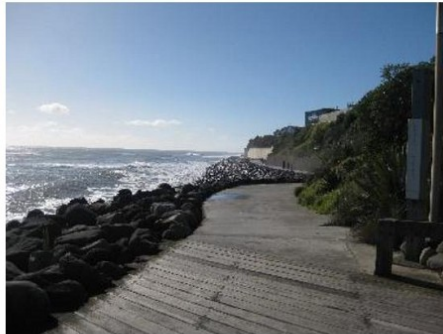
Water front walkway in New Plymouth New Zealand where sea washes over the natural timber, along with and continuous salt spray attacks the timber as shows signs of dry rot, splitting, and general corrosion to fittings.
