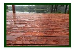
As the lanolin dries the natural waxes are absorbed into the timber. This sets up a protective barrier so water will bead and not penetrate the timber.
