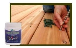
When building new timber decks use Lanolin Grease LG100 to coat the screws and nail to lubricate them and protect them form corroding internally. It also protects the wood internally from water ingress through the screw/nail holes.
