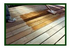
Apply using a fine mist spray or lambswool applicator. One coat is usually sufficient but if the wood is still dry further coats can be applied after a minimum of 6 hours. (able to be walked on within 24 hours)
